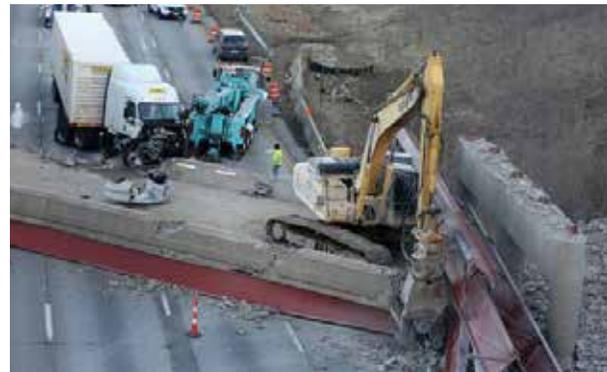
**University of Cincinnati** architecture professor Tom Bible said the pictures indicate a failure of the joints at the western joint of the span. That wouldn't have happened, he said, if the eastern end of the bridge over the median and connecting to the old Hopple Street connection hadn't been previously removed. "Judging from the pictures, it obviously slipped off its supports," he said.
